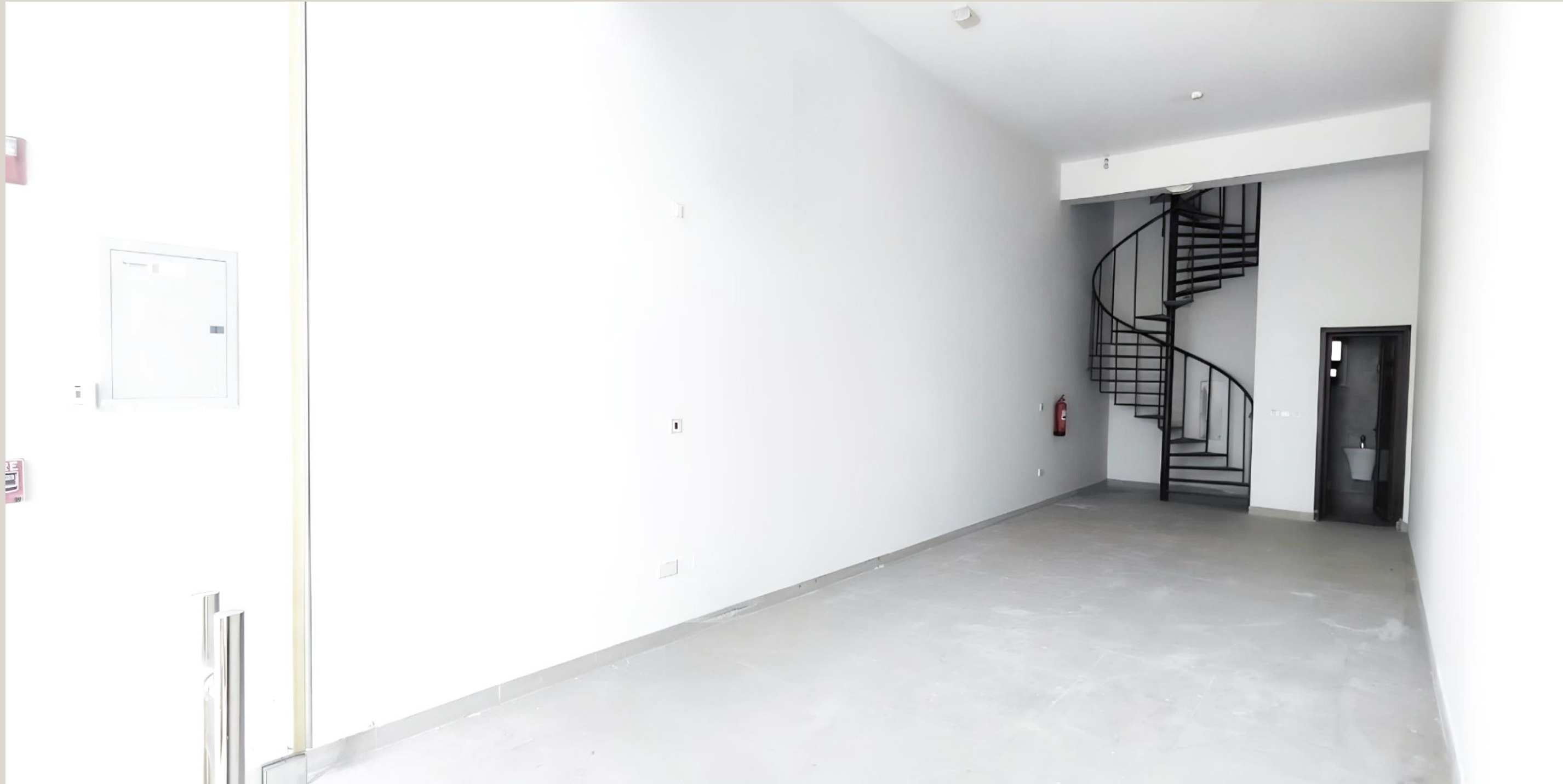
Ground Area Actual View
